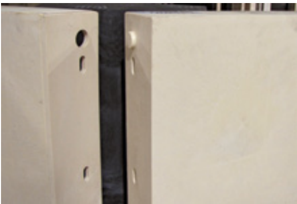
VIEW OF ALIGNMENT TABS AT TOP OF KAFKO POLYMER PANEL
